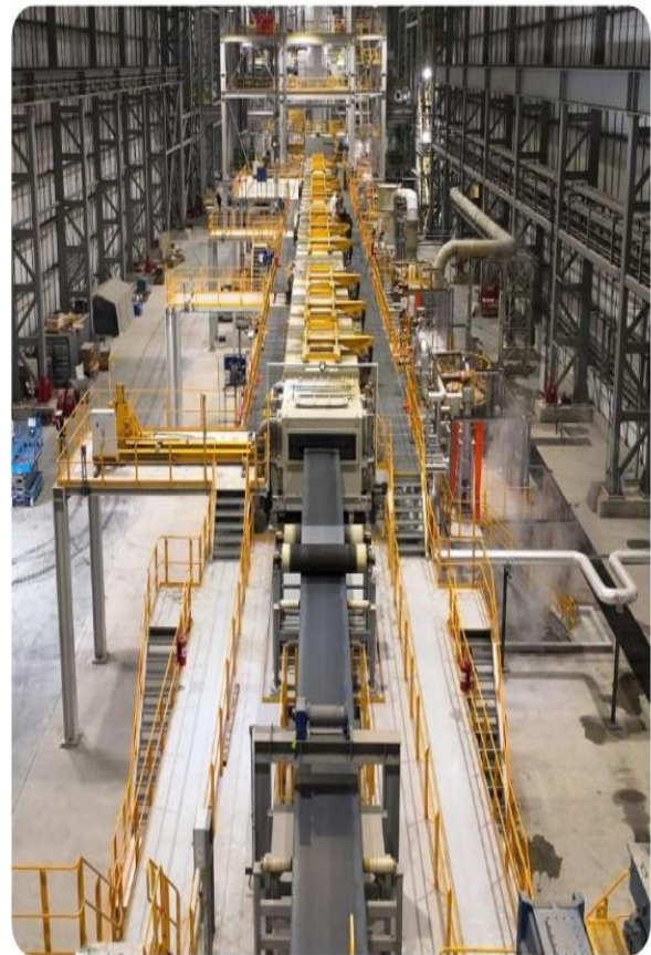
Pickling and Galvanizing Line
