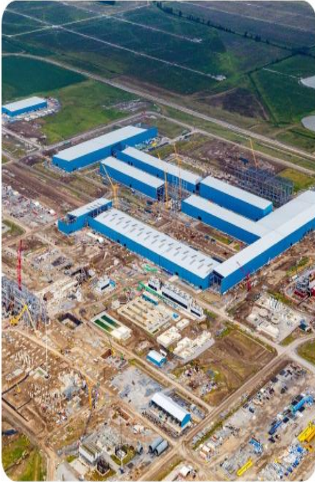
Aerial View Big River 2
