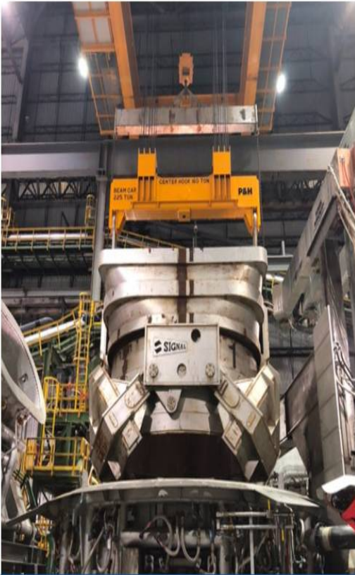
Electric Arc Furnace at Fairfield Tubular
