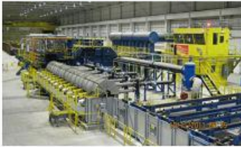
Lorain #6 Heat Treat & Finishing Facility
