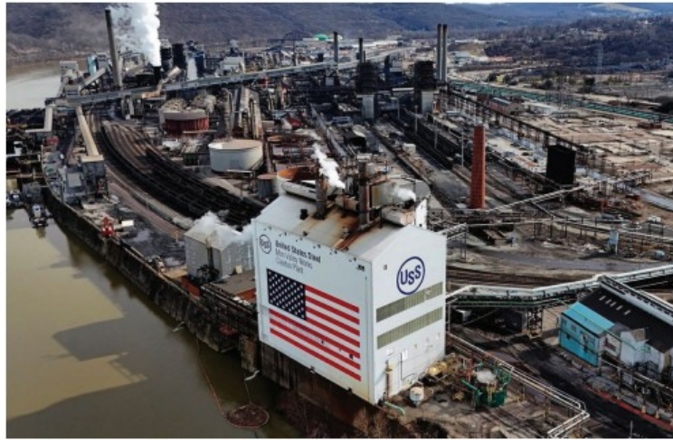
The United States Steel Mon Valley Works Clairton Plant in Clairton, Pa., is shown on Monday, Feb. 26.
